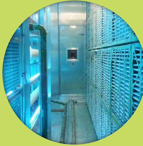
Induction of MERV 13 Filters & UVGI. to AHU's
